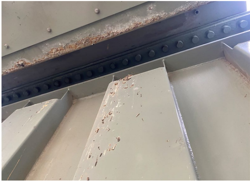
Plate 10: Bird Droppings Within Transformer
