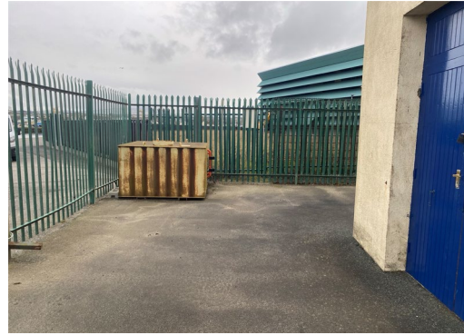
Plate 2: Built-up Area Surrounding Substation
